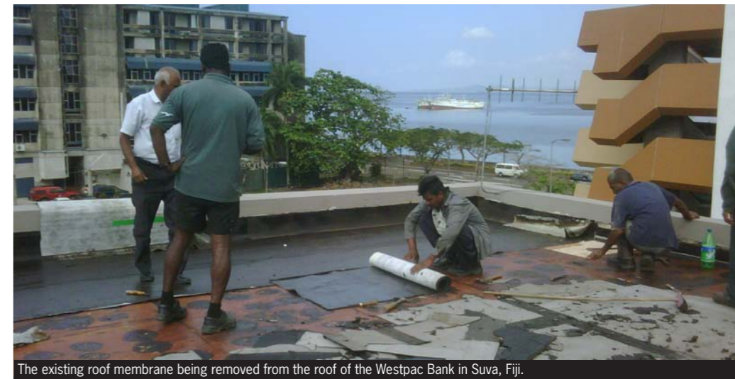
The existing roof membrane being removed from the roof of the Westpac Bank in Suva, Fiji.
