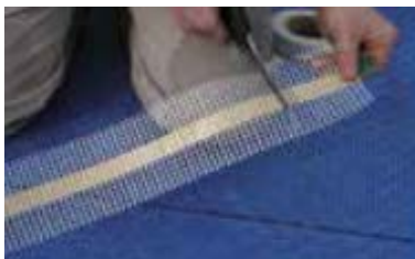
7. Install overlay tapes
