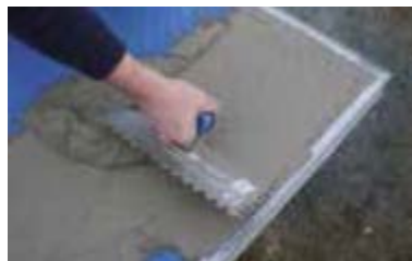
8. Commence with tiling, using ARDEX X18+/-E90 or ARDEX X77+/-E90
