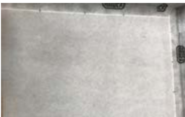
4. Apply ARDEX STB tape to form overlap on all external drainage profiles
