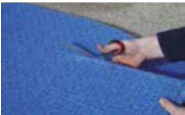
6. Measure and cut the mat to achieve the correct fit.
