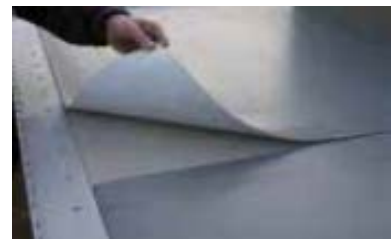
5. Install WPM 1000 to balcony as per ARDEX technical literature
