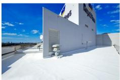
Specifications required a new membrane that could be installed over the existing membrane – to negate the need for removal of the existing membrane (a process that would present an element of risk to guests and employees of the resort). The membrane would also have to be able to withstand high wind speeds, consistent with its Zone B grading, while contributing to the ongoing reduction in energy consumption.
