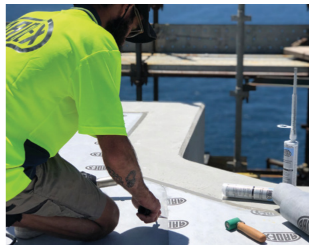
Coastal Penthouse Flat Roof – East Coast
