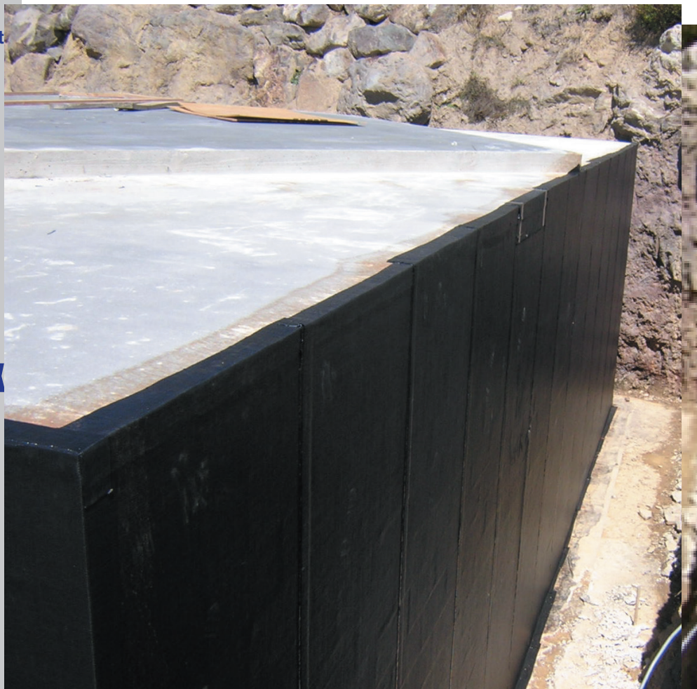
Typical waterproofing using Shelterseal 3000X
