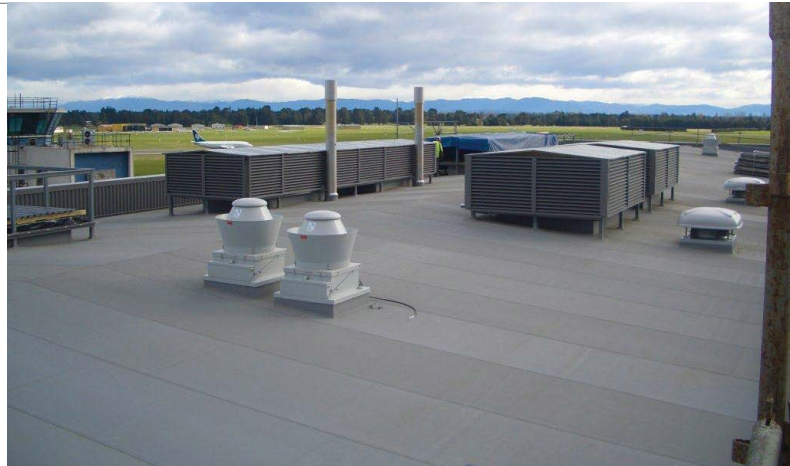
The new Christchurch Airport Terminal has been covered with 1.5mm Dove Grey Butynol.
