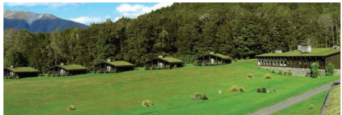
The chalets at Takaro Lodge, Te Anau are an early example of living roofs using ARDEX Butynol as a waterproofing membrane. Completed in 1970.
