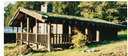
The chalets at Takaro Lodge, Te Anau are an early example of living roofs using ARDEX Butynol as a waterproofing membrane. Completed in 1970.
