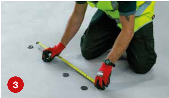
3 Apply correct fasteners for the application at centres determined by a Wind Load Calculation, if required.
