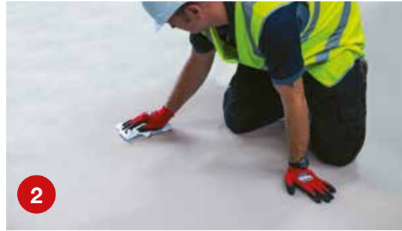
2 Clean surface with appropriate solution as recommended by the membrane manufacturer.
