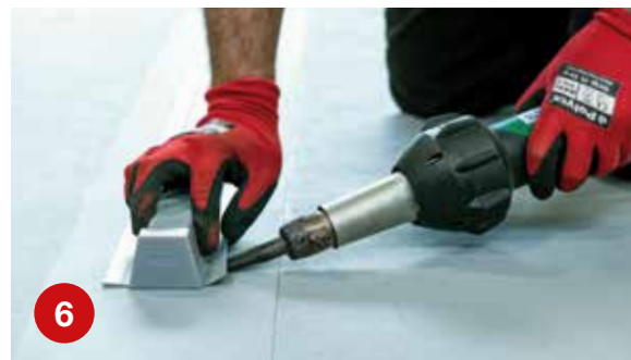
6 Hot-weld 'EJOBAR TPO 2G' in the centre of the membrane, directly over the line of fasteners.
