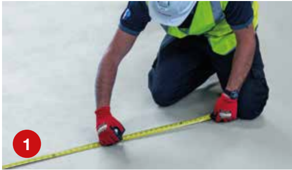
1 Accurately measure and mark out the 'EJOBAR TPO 2G' installation area.
