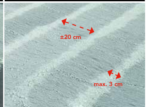
Optimal spray width should be +/- 20 cm, with max. 3 cm overlap between spray lines.
