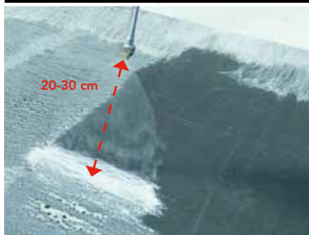
The optimal distance from the spray gun nozzle to the surface should be 20 - 30 cm.
