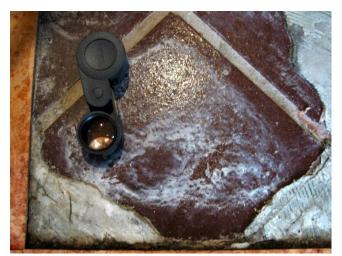
Ceramic tiles which were covered with ARDEX K15. The glaze and other residues were not fully removed prior to the application of the levelling cement was partially responsible for the Neoprene primer to de-bonding. Also this location had rising damp (white efflorescence on the tile) which further degraded the K15 and loosened the primer bond. Vinyl tiles debonded off the floor.
