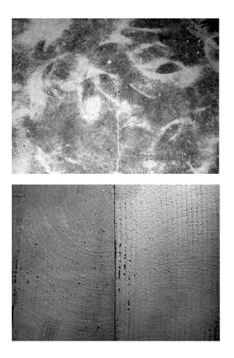
A concrete floor coated with a curing compound. The floor has been partially ground, but not sufficiently to promote good adhesion.
