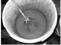
The ARDEX mixing paddle, and mixing of material with the paddle and a heavy duty drill.
