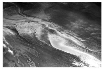
This floor shows shrinkage related cracks due to product installation problems.
