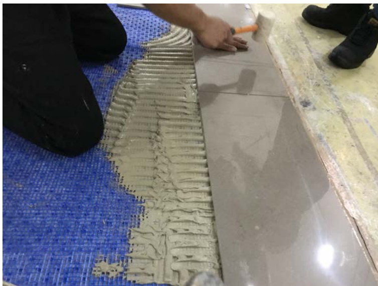
Figure 1.6: Installation of tiles
