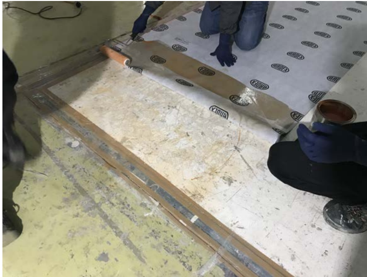
Figure 1.3: Installation of waterproofing layer ARDEX WPM 1000
