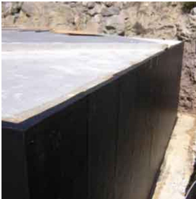
Typical waterproofing using Shelterseal
