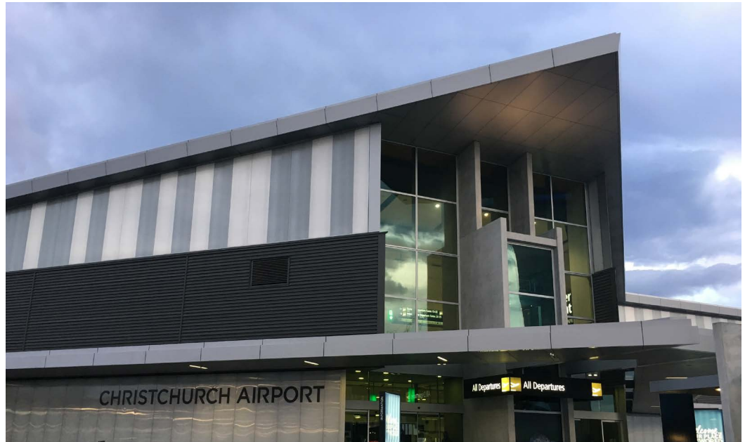
Christchurch International Airport 4500 m 2 of 1.5 mm Grey Butynol used for flat roof areas and gutters. Completed in 2013.
