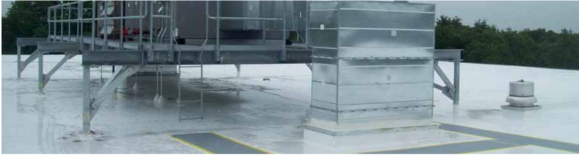
Picture 1.11 - Walkway protection
