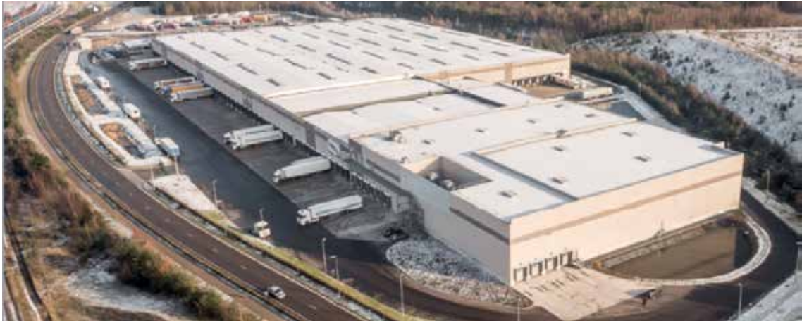
Picture 1.5 - Lidl distribution center - Genk, Belgium
