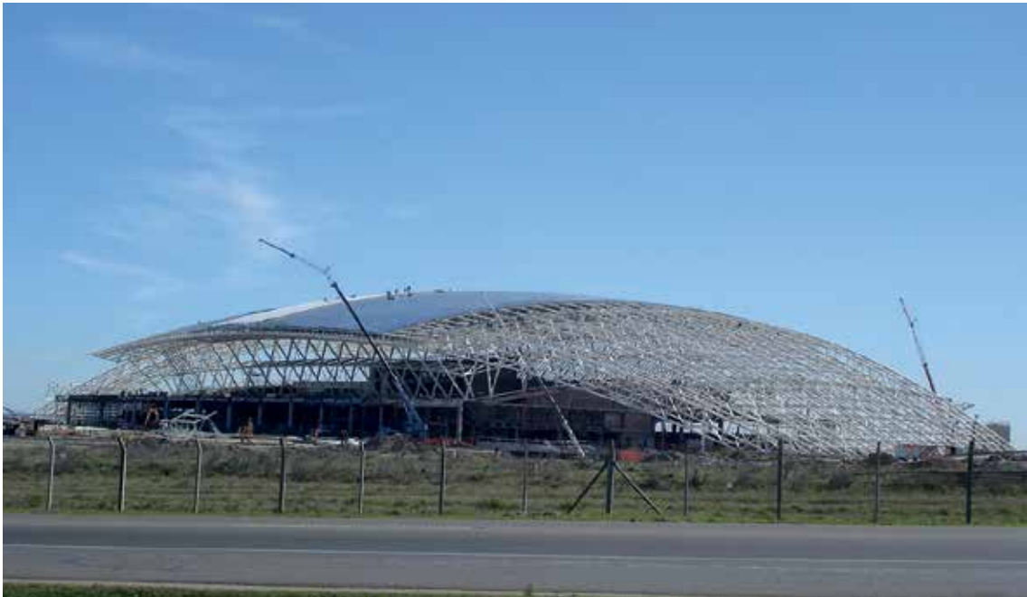
Picture 1.13 Construction airport terminal - Montevideo, Uruguay
